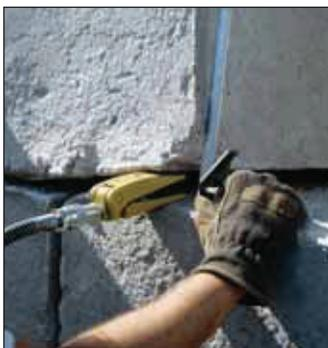
◀ A **WR-5** wedgie cylinder is used to position a concrete block on a construction site.
