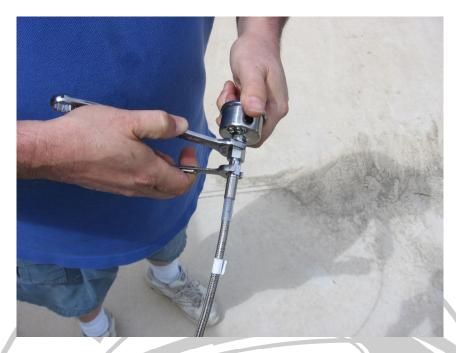
Thread the hose to the fitting on the gauge; use a 9/16 wrench on the gauge fitting and a 7/16 wrench on the hose fitting to tighten.
